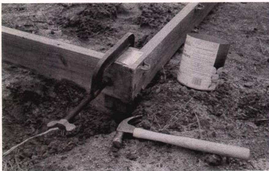
Figure 4. Foundation side and end boards are attached to 4-by-4 posts to anchor the structure. Note the EMT clamps on the side boards hold the PVC pipe ribs.
